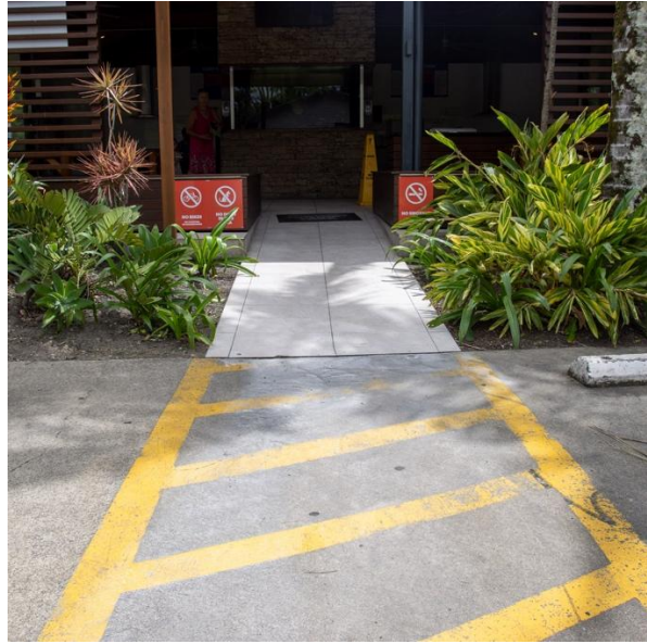
The ramped access to the camp kitchen.
