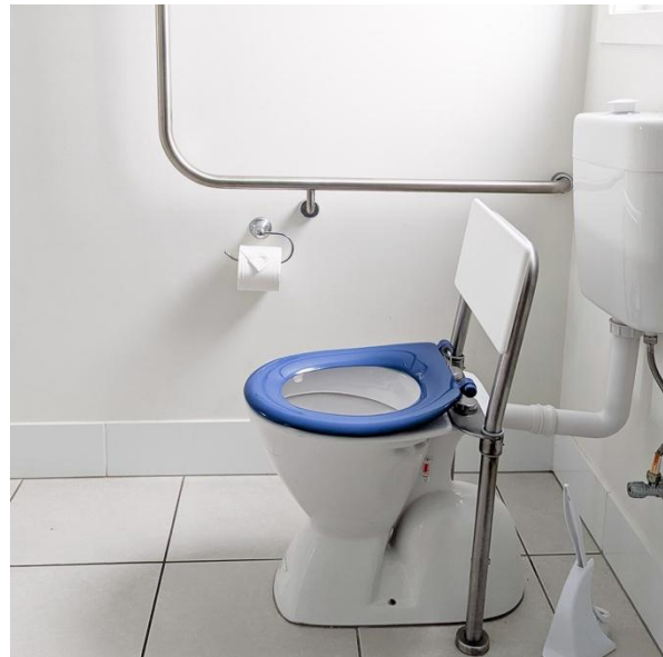
The accessible toilet is right hand transfer with grab rails.
