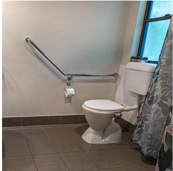
The toilet has a right-hand-side transfer with grab rails along the wall.
