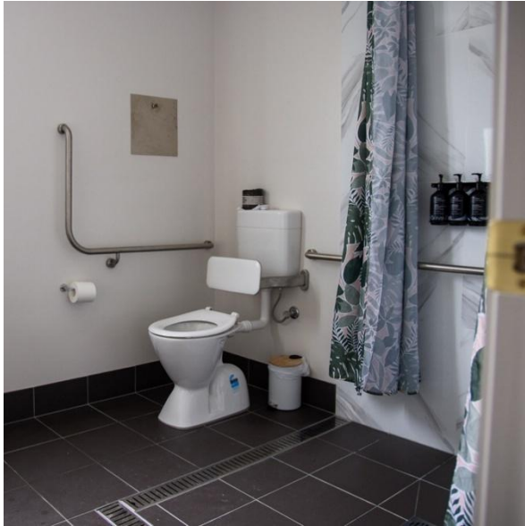
The accessible bathroom has grab rails across the side and back of the toilet pan.
