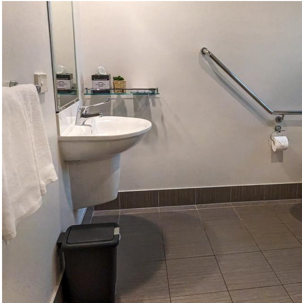
The accessible bathroom has leg clearance under the basin and a lever-style tap head.
